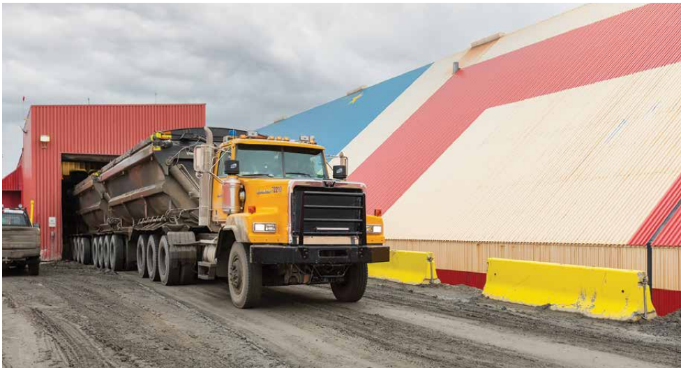
Teck innovated the air wash system that removes dust from trucks as they exit the Truck Unloading Building.
