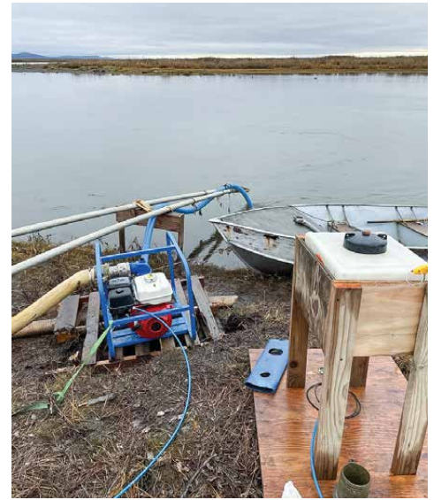
Kivalina's community water fill location in the Wulik River in September, showing the updated pump and hoses provided by Teck.
