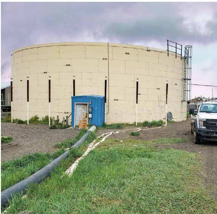
The community of Kivalina must fill their water storage tanks in the summer months, so they have enough water to make it through the winter.
